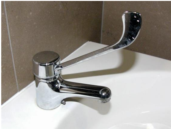
Figure 29 - The photograph shows a single lever mixer tap which can be easily used by a large number of persons regardless of their motor abilities.
