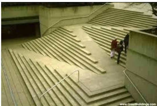
Figure 28 - The photograph shows an example of universal design, a stair/ramp - "Stramp" - designed by Cornelia Oberlander and Arthur Erikson. The stair/ramp is situated in Vancouver, and is accessible to everyone ( http://accessibility-fail.dreamwidth.org/1101.html ).
