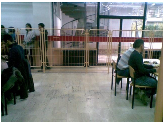
Figure 26 - An example of bad practice: The photograph shows a student cafeteria in which a partition wall hinders access and maneuvering.
